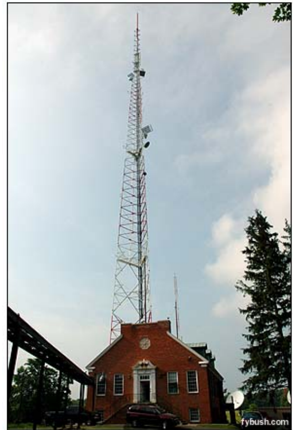
The building and WFSB's tower
