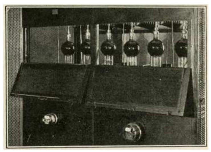
Six mercury vapor type tubes in a series circuit are used in the 350KW Rectifier
