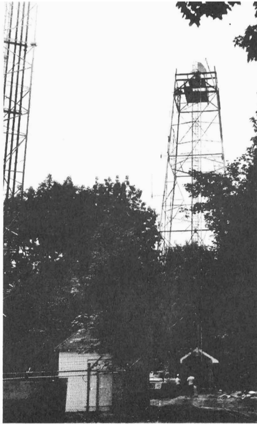
Fig. 3 Radar RF system at Avon, Conn. The radome had not been installed when this picture was taken.
