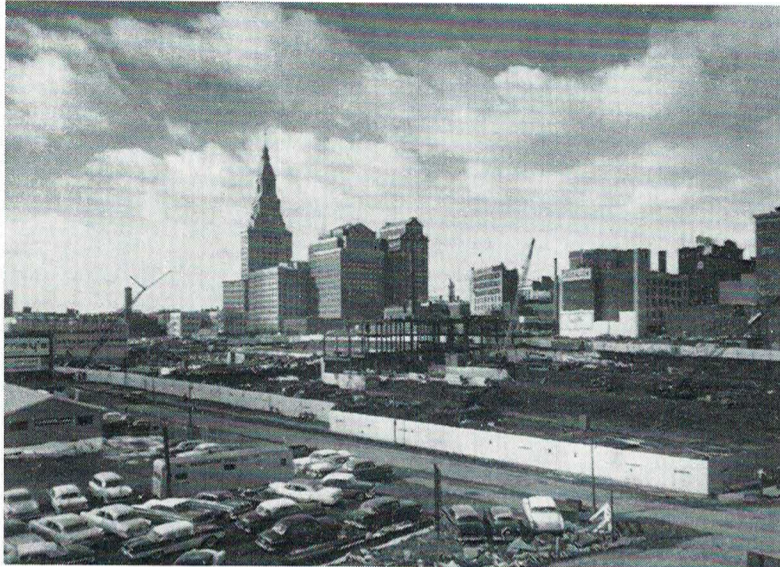
A BIRD'S EYE VIEW of Constitution Plaza, with The Travelers Home Office group of buildings in the background, shows steel on the rise for a new bank and office building and, to the far left, a part of Broadcast House, new home of The Travelers Broadcasting Service Corporation.
