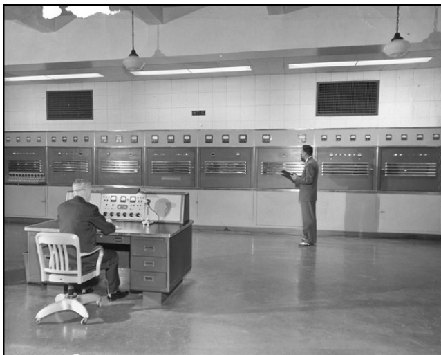
The Westinghouse 50HG-1 fifty-kW transmitter purchased in 1947 to replace the original 50-kW RCA transmitter. (From hardfordradiohistory.com.)
