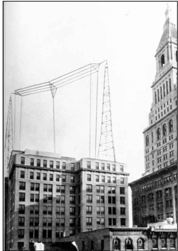
Two towers on the roof of the company's Grove Street building supported a "flat-top" or T-shaped wire antenna, commonly used at the time.
