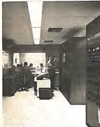
WTIC Radio's Master Control room, shown here, is the heart of the technical operation. All lines terminate here and the sound from all studio amplifiers must pass through the equipment shown prior to feed to Avon Mountain transmitting site.
