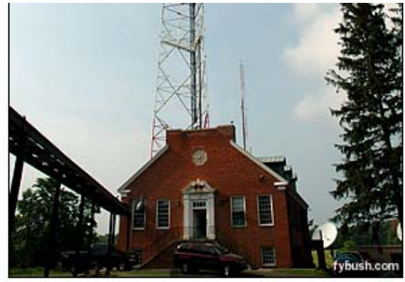
The building and WFSB's tower
