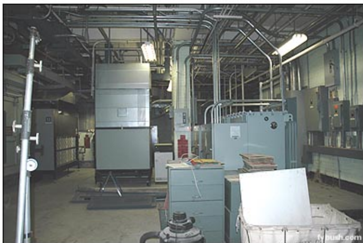
Down in the basement
